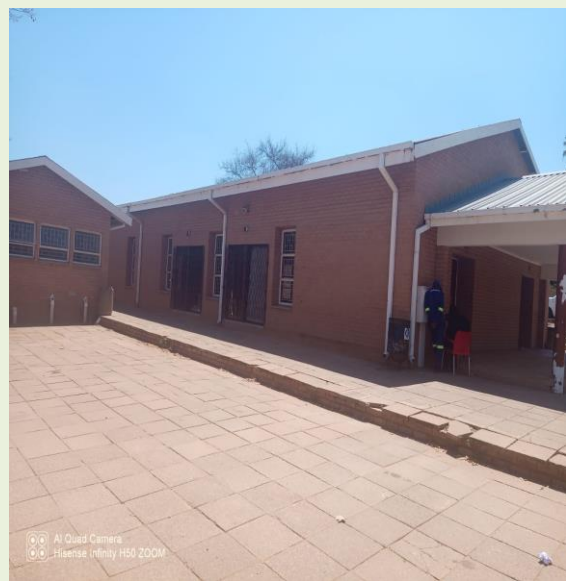
FIGURE: 4 JINNAH PARK COMMUNITY HALL
